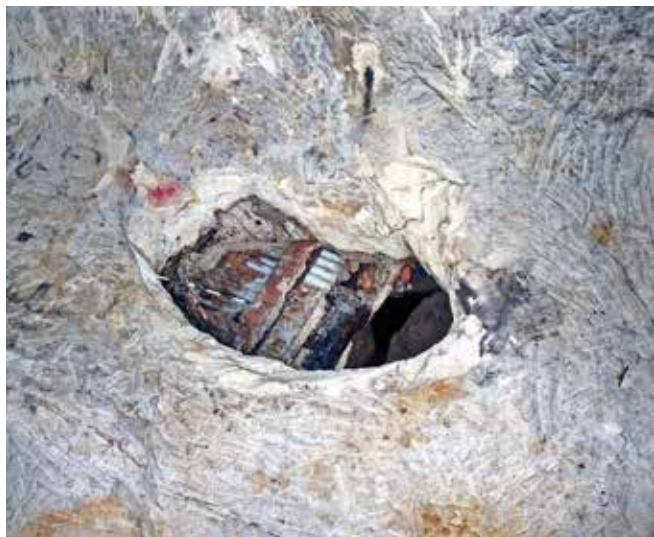
The collapse in the floor of Barons Cave looking down into the Auction Room mine below in May 1987
